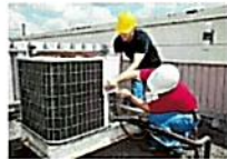
Commercial Rooftop Replacement
