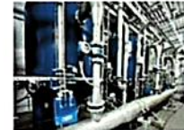
Boiler, Chiller & Central Plant Upgrades
